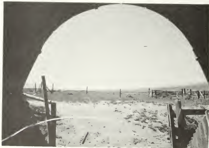
Looking South from Pipe; note fencing as compared to opposite entrance.
